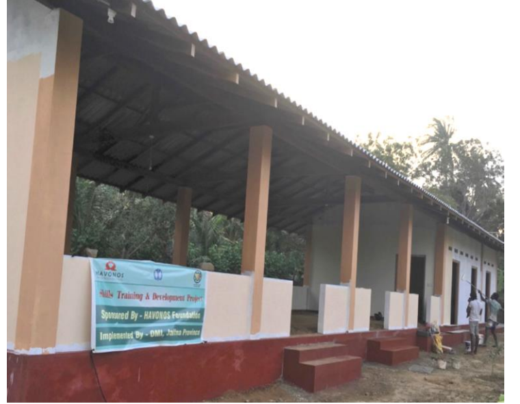
Classrooms nearly completed
