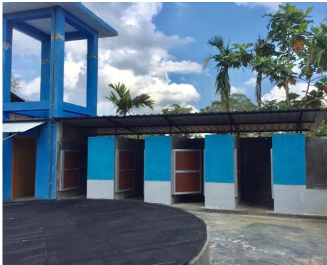
New showers with well and water tank
